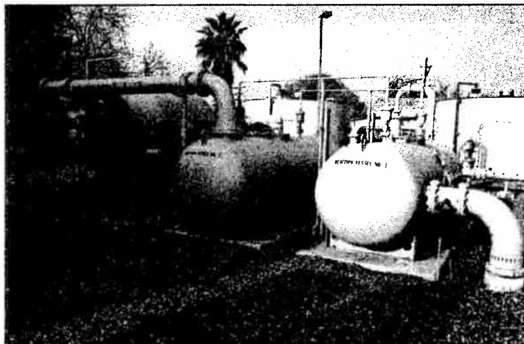
Photo 1 – Typical Filtronics filter vessel (behind blue & red piping) and reaction vessels. Note sodium hypochlorite chemical oxidant injection point (foreground right) and backwash reclamation tank (right background).
